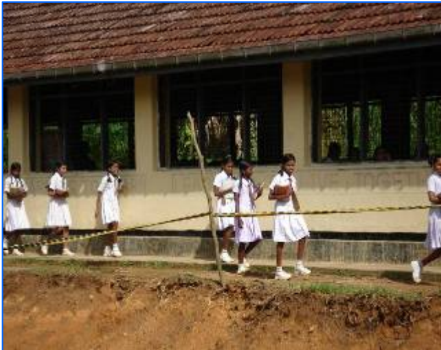
Landslide affected school in Ratnapura district
